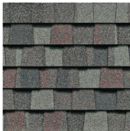
ROOF Colonial Slate
